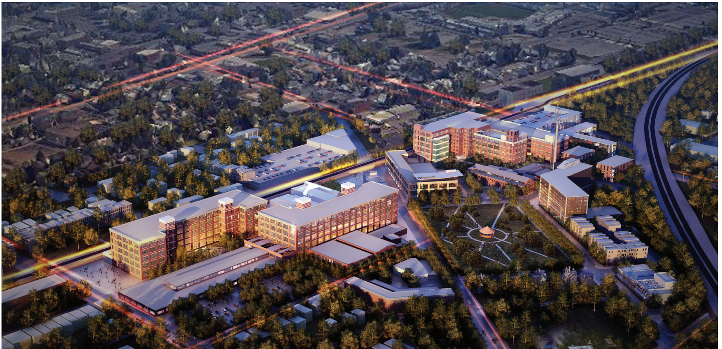
Electric Works, Fort Wayne, Indiana
